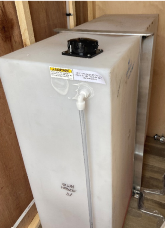
On-Board Freshwater Tank Showing Fill Cap And Water Level Sight Tube
